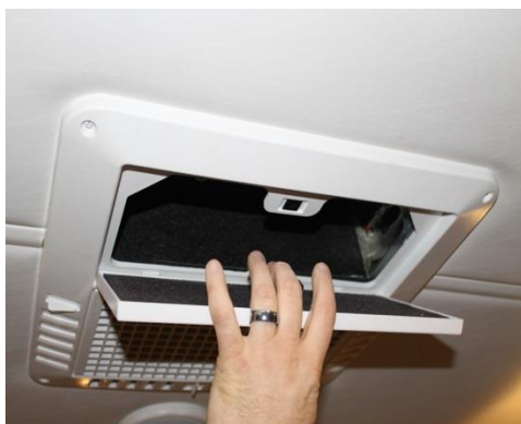
Removal of A/C filter
