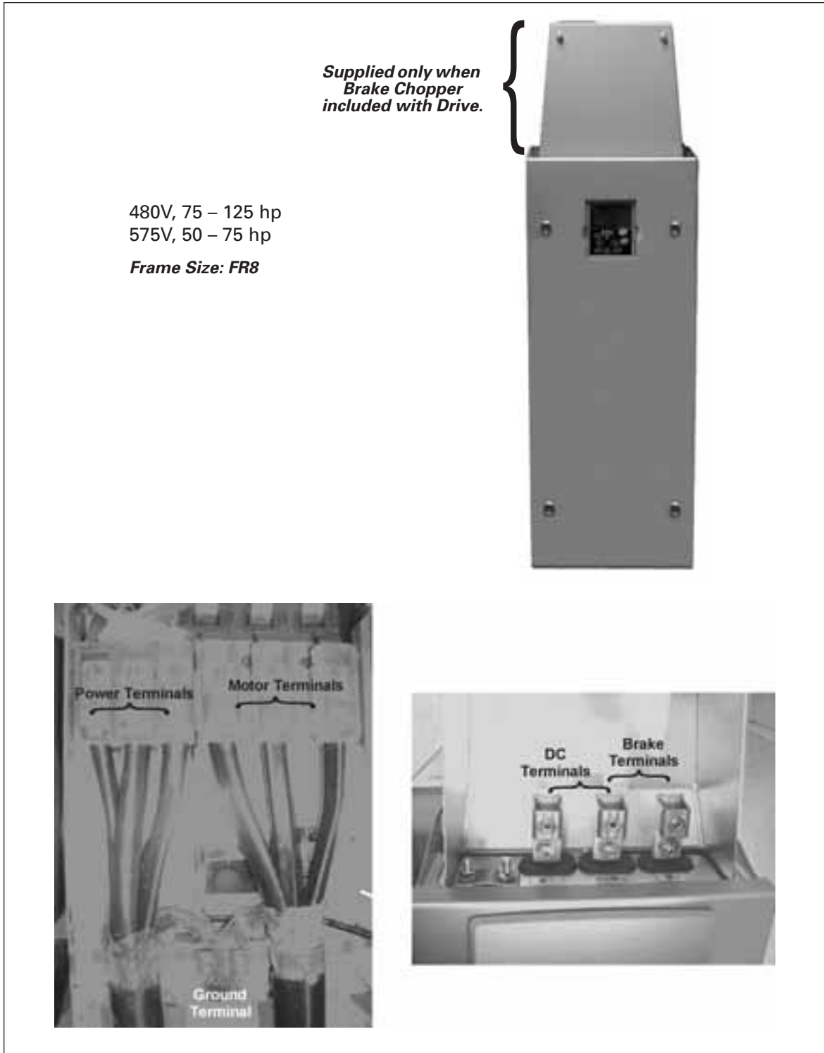
Figure 3-12: FR8 Power and Motor Wiring Terminals
