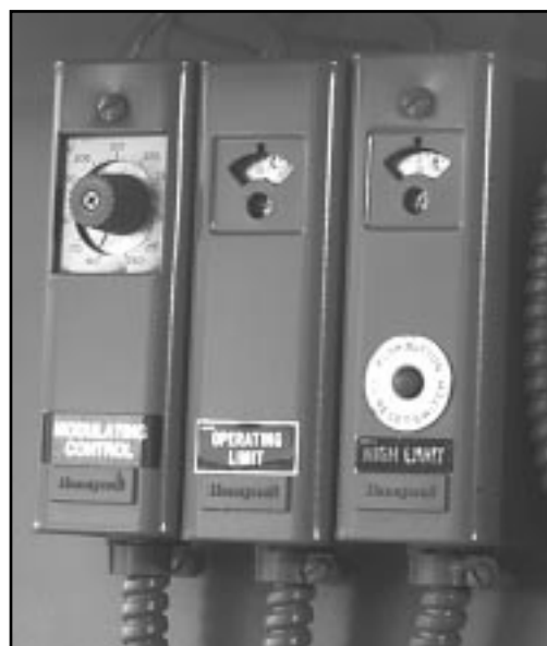
Figure: 6-5 Hot Water Controls
