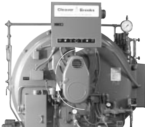
Figure: 5-3 Fan Motor and Air Pump, Clockwise Rotation (CB)
