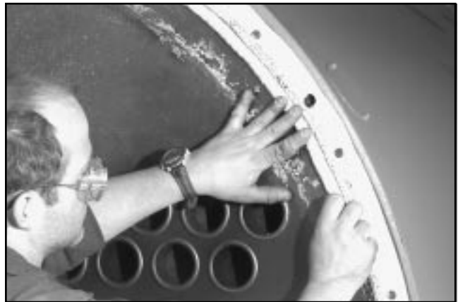
Figure 8-29: Rope Gasket Glued against Tadpole Gasket
