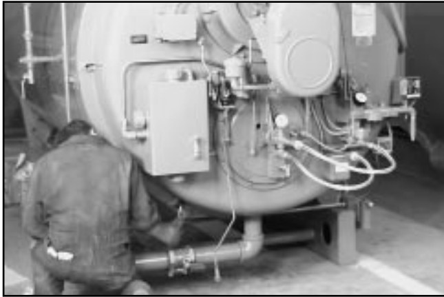
Figure 8-35: Close and Tighten Front Head
