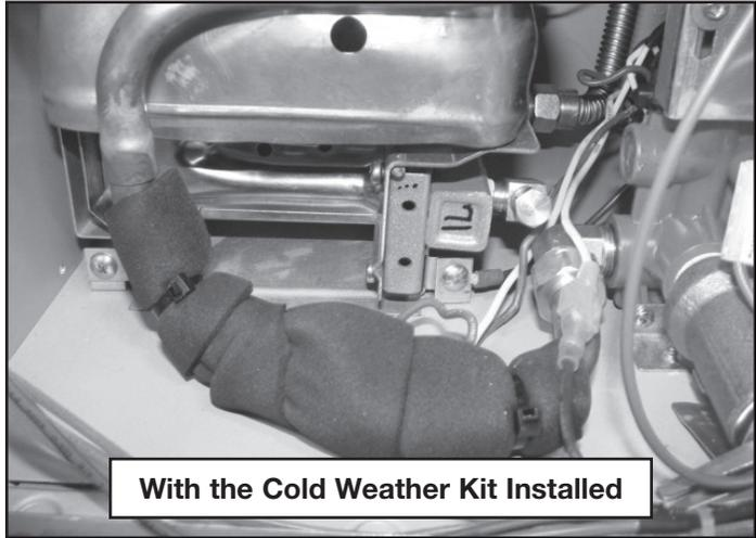
**With the Cold Weather Kit Installed**
