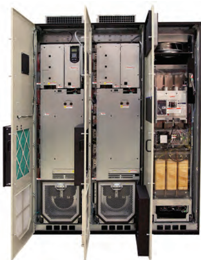
IP54, NEMA Type 12 Drive and Options (2500 MCC Style Cabinet) (Frame 9 shown)
