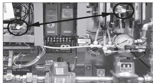
FIGURE 19.2 – HIGH & LOW-PRESSURE TEST PORTS
