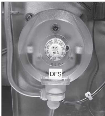
FIGURE 22.2 - DIRTY FILTER PRESSURE SWITCH
